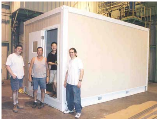
Climate Chamber Under Construction
