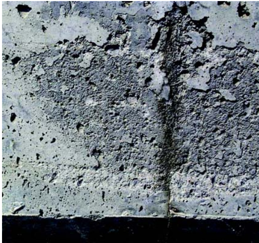
Figure 9. Scaling of concrete
