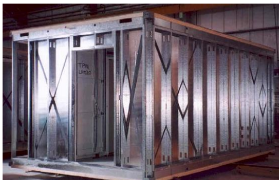
Figure 2. Wall-Load Bearing module with steel C-section profiles (Lawson et al., 2005b)
