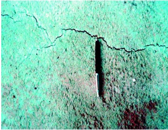
Figure 7. Plastic shrinkage cracking
