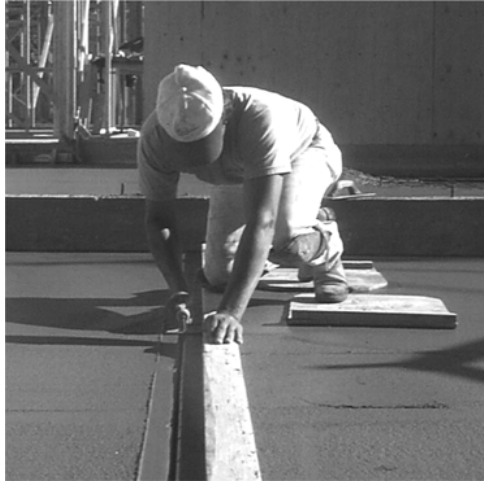
Figure 1. Grooving of concrete slab
