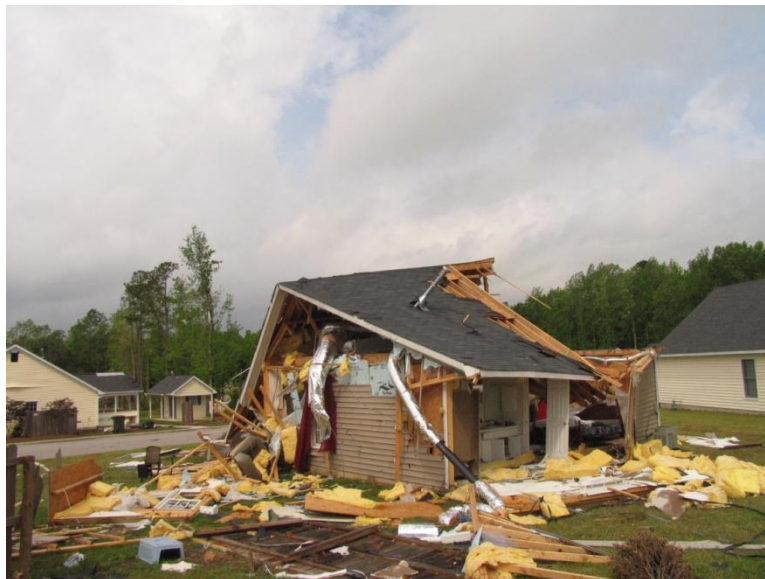
Figure 4 – Envelope Failure of Foam Sheathed Exterior Walls
