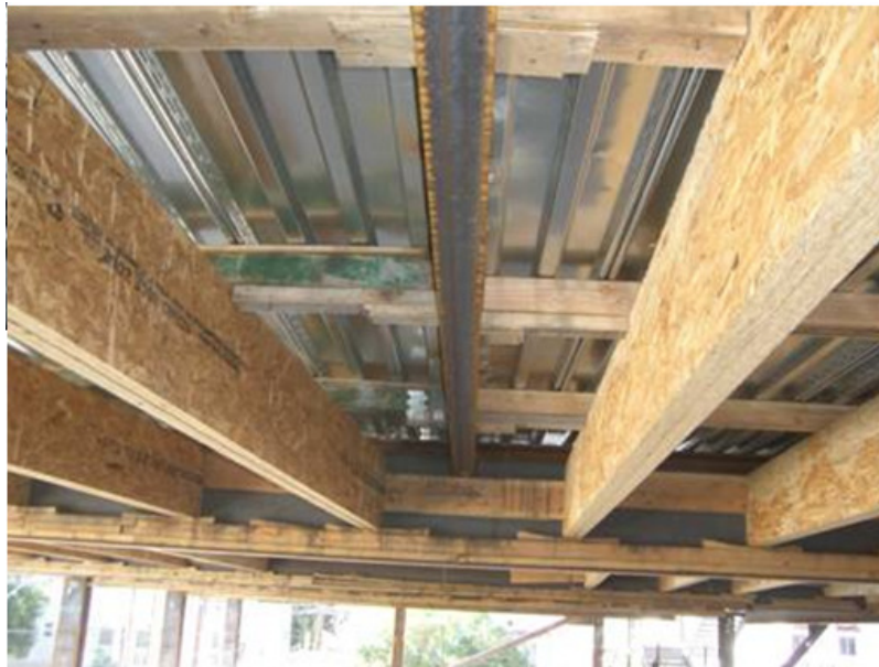
Figure 4: Self Shoring System In Place
