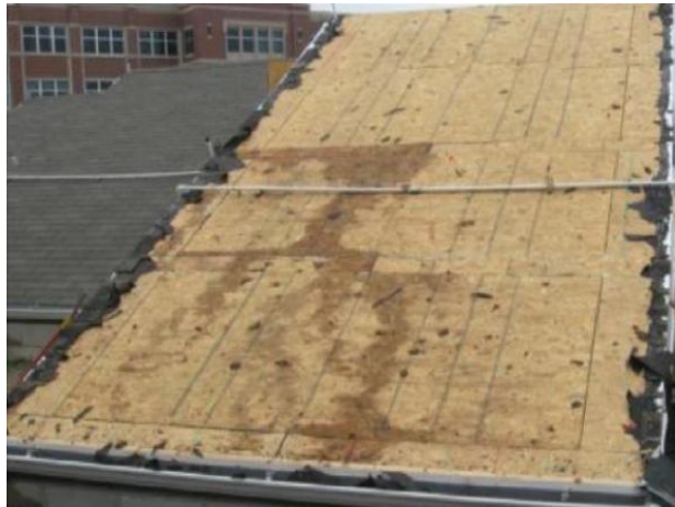
(a) Moisture Buildup in Sheathing
