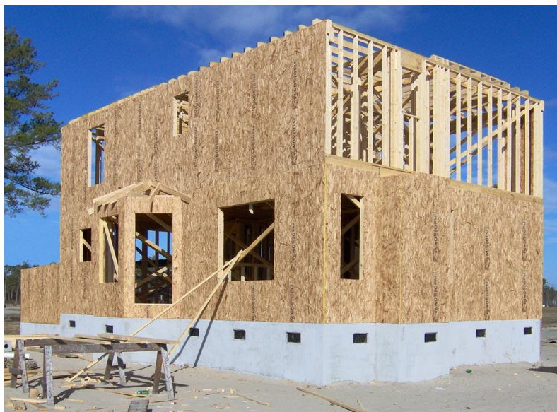
Figure 7 – With thoughtful layout, continuous structural sheathing can resist both shear and uplift forces, providing cost-effective continuity between the foundation and roof framing connections. Oversize panels may be used to eliminate blocking by locating horizontal panel joints at the rim joists and to match the dimensions of taller wall systems.
