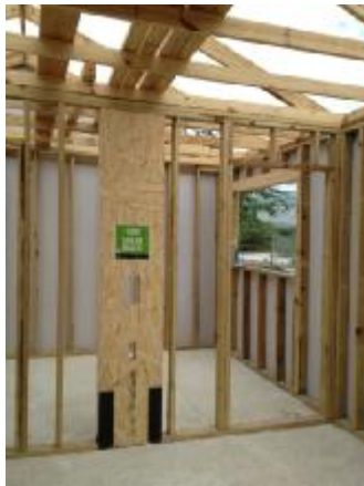
Figure 9. TJ-Shear Brace at interior braced wall location.
