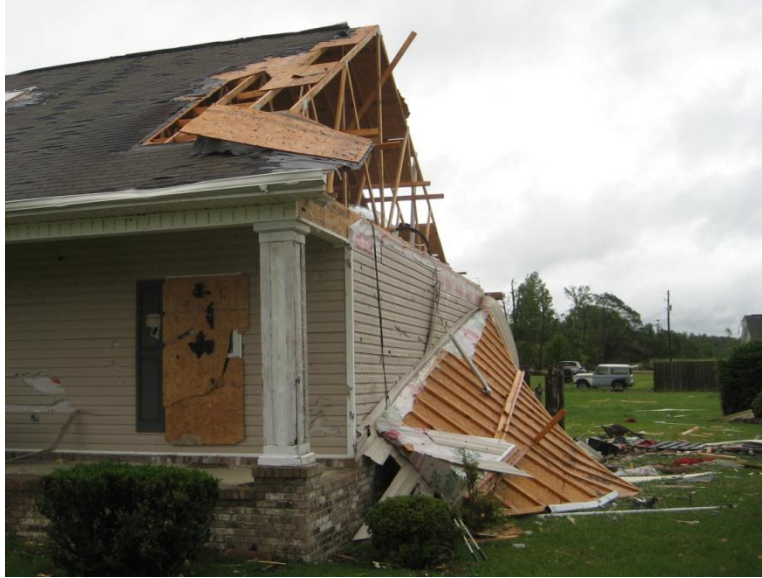
Figure 5 – Failure of Gable-end Framing.
