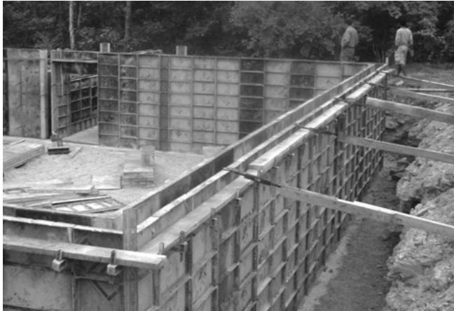
Figure 5. Metal framework with plywood sheathing faces
