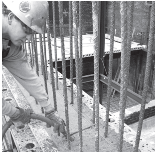
Figure 3. Vibration of concrete
