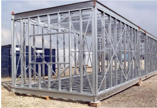
Figure 6. Corner-Supported module (Lawson et al., 2005b)
