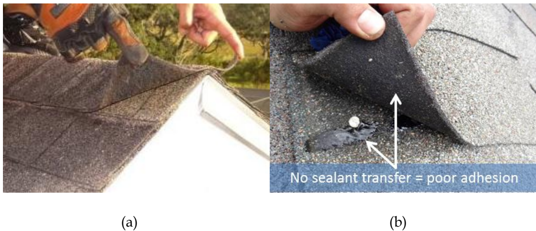
Figure 6. Typical unsealed ridge and hip cap shingle conditions: (a) no sealant strip below cap and (b) poor adhesion on edges of cap.
