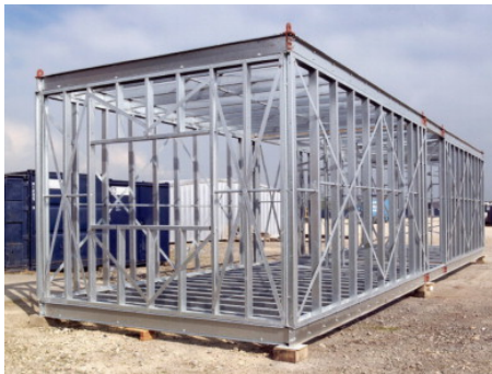
Figure 2. Corner Supported 3D Module (image by Lawson and Ogden, 2008)
