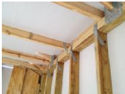
Figure 10. Typical uplift connections.
