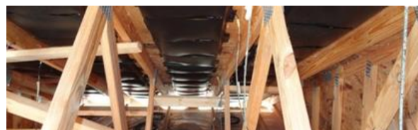
(b) Air Gap Prior to ccSPF Installation
