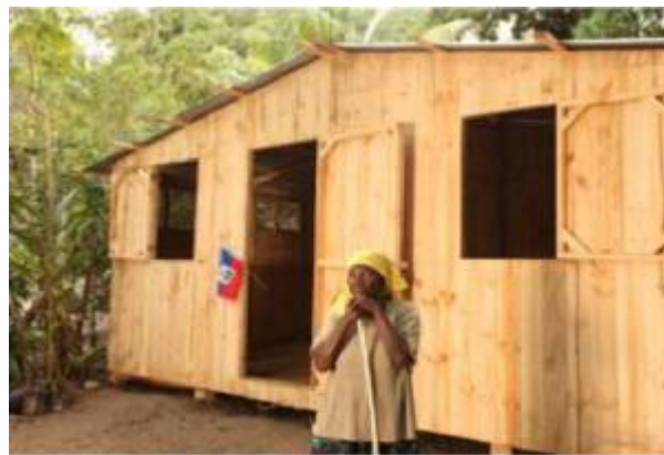
Figure 2. UTPMP transitional shelter.
