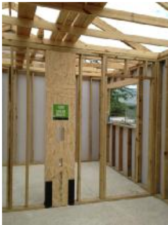
Figure 9. TJ-Shear Brace at interior braced wall location.
