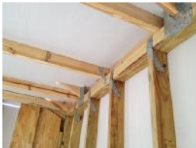
Figure 10. Typical uplift connections.
