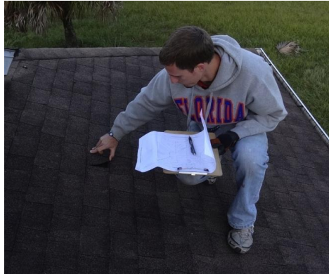
Figure 2. Partially unsealed field shingle discovered during a survey.
