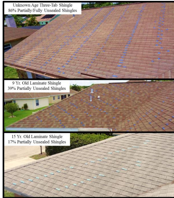
Figure 3. Patterns of partially/fully unsealed three-tab and laminate shingles. (Note: blue tape denotes location of unsealing).
