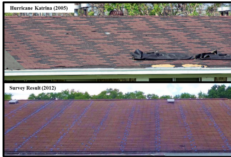
Figure 8. Potential link between (top) post-hurricane Katrina damage observed by FEMA (2012) and (bottom) observations of pre-existing unsealing during roof surveys.
