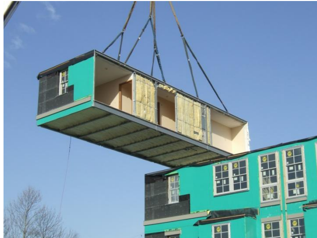
Figure 1 - Placement by crane, top pick
