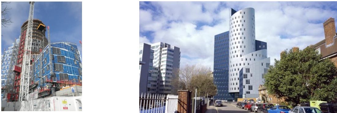
Figure 6. Concrete core construction Victoria Hall, UK ; Core visible on left, rendering of completed structure on the right (images by MBI, 2013a)
