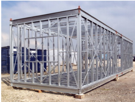
Figure 2. Corner Supported 3D Module (image by Lawson and Ogden, 2008)
