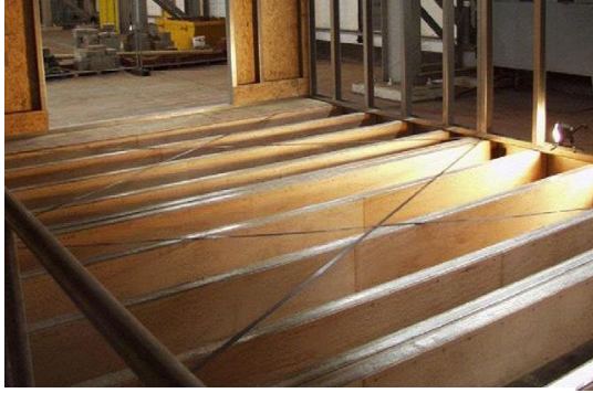
Figure 4. Individual module diaphragm of a module (Lawson et al., 2008)
