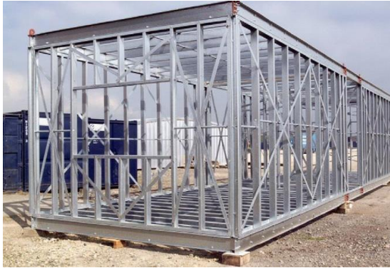
Figure 6. Corner-Supported module (Lawson et al., 2005b)
