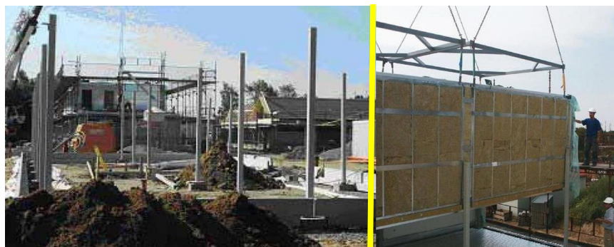
Figure 8. Two photos from two different stages of construction of an Openhouse building (Bengt Birgersson, 2004)
