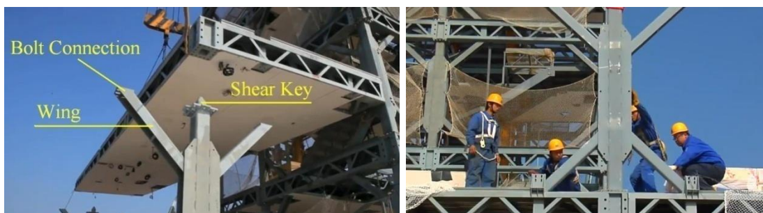
Figure 1. Dongting Lake Hotel with 2D structural system using floor cassette-column-connection example (Jackson, 2012)
