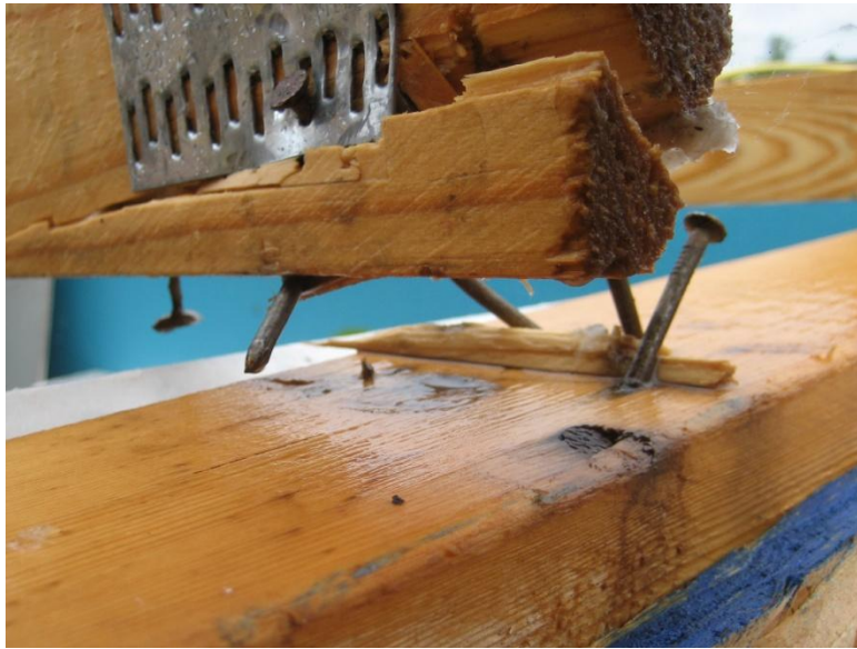
Figure 2. Toe-nailed Connection of Roof Framing-to-Wall.
