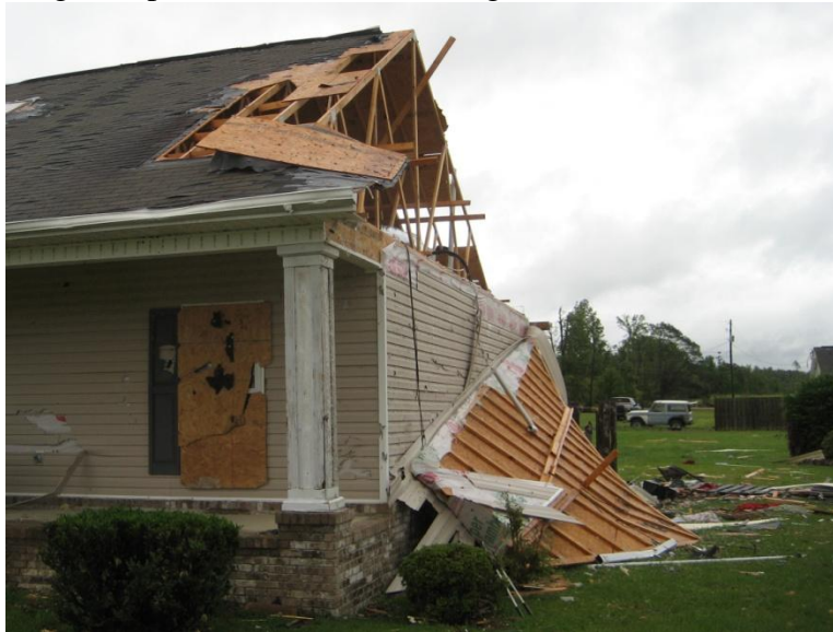
Figure 5 – Failure of Gable-end Framing.
