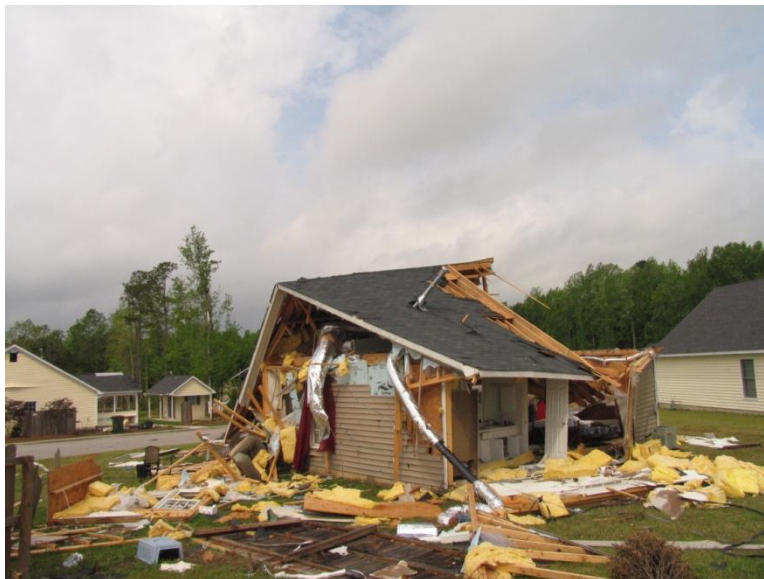
Figure 4 – Envelope Failure of Foam Sheathed Exterior Walls
