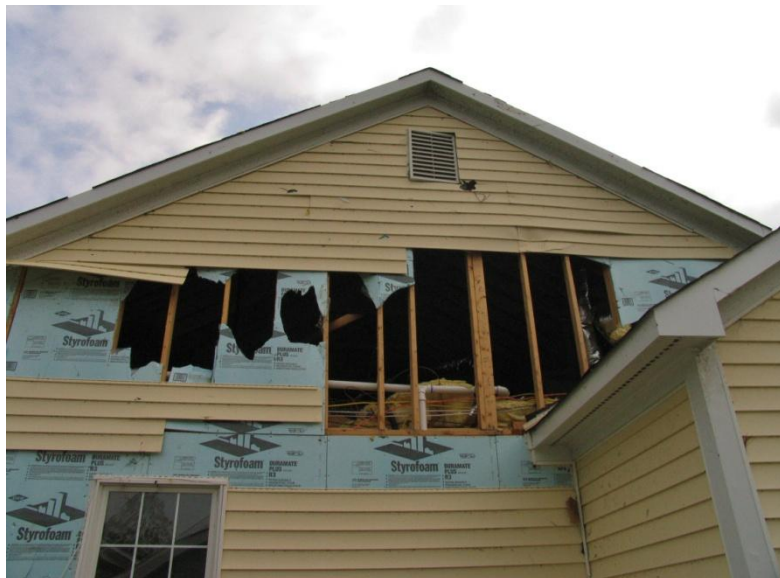
Figure 6 – Non-Structural Sheathing at Gable-end after minor wind event.
