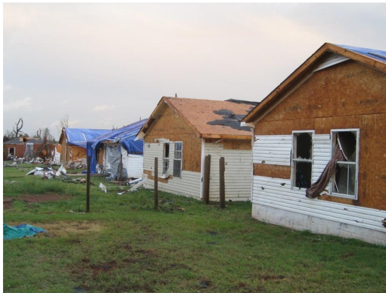
Figure 1 –Building Envelopes Fully Sheathed with Wood Structural Panels.
