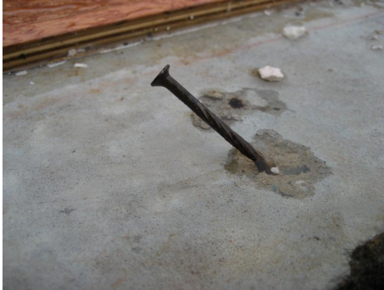
Figure 3 – Failed Nail Connection of Wall Bottom-Plate to Slab.
