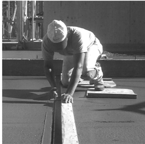
Figure 1. Grooving of concrete slab
