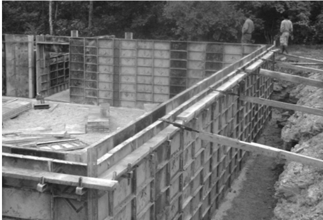
Figure 5. Metal framework with plywood sheathing faces
