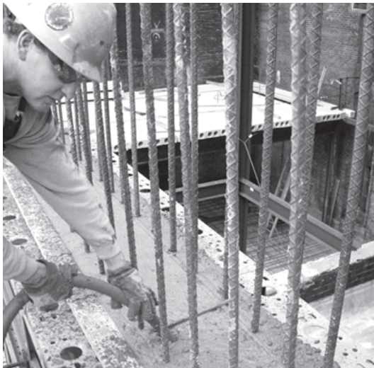
Figure 3. Vibration of concrete
