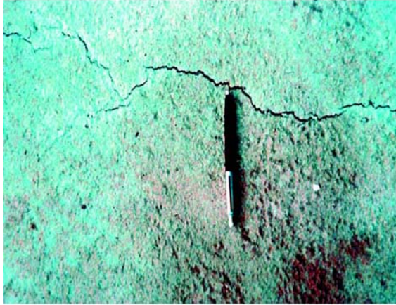
Figure 7. Plastic shrinkage cracking
