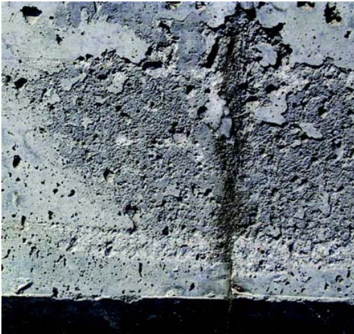
Figure 9. Scaling of concrete
