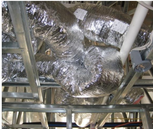
Poorly installed ducts
