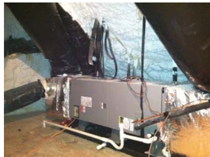
Alternative: Insulation at the roof deck
