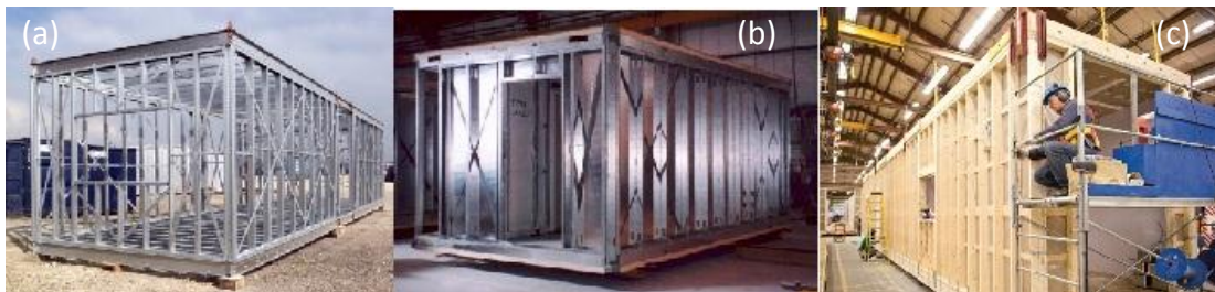
Figure 3. (a) Corner-post bearing module (image by Lawson and Ogden, 2008), (b) CFS wall bearing module (image by Lawson and Ogden, 2008) (c) Wood wall bearing module (image by Modular Building Institute)
