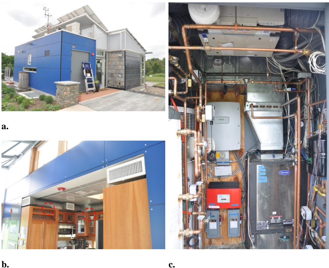
Figure 3. a. MorningStar Solar Home; b. Two of four measurement locations near duct diffusers; c. Packaged unit in mechanical room; red dots are approximate locations for \frac{1}{2} in. diameter traverse caps to be installed in the ductwork to enable velocity profiling and to fit particle injection line
