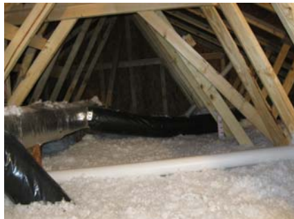
Default: Insulation at the ceiling
