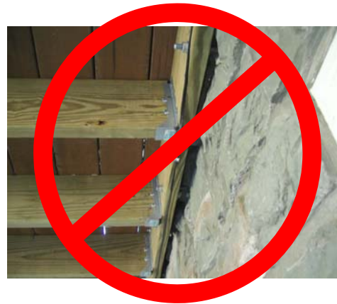
Figure 17. No Attachment to or Through Exterior Veneers (Brick, Masonry, Stone)
