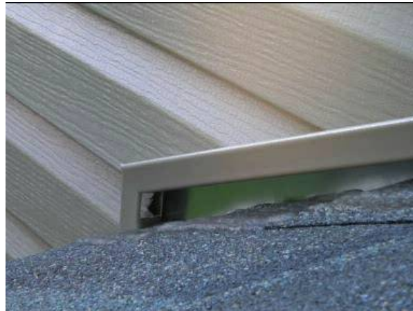
Missing step & kick-out flashing
