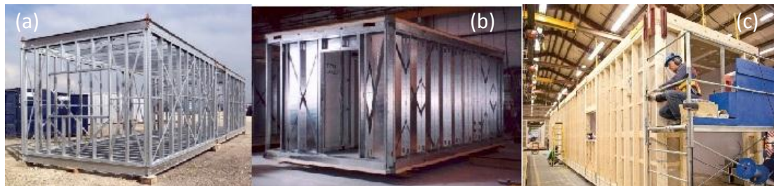
Figure 3. (a) Corner-post bearing module (image by Lawson and Ogden, 2008), (b) CFS wall bearing module (image by Lawson and Ogden, 2008) (c) Wood wall bearing module (image by Modular Building Institute)
