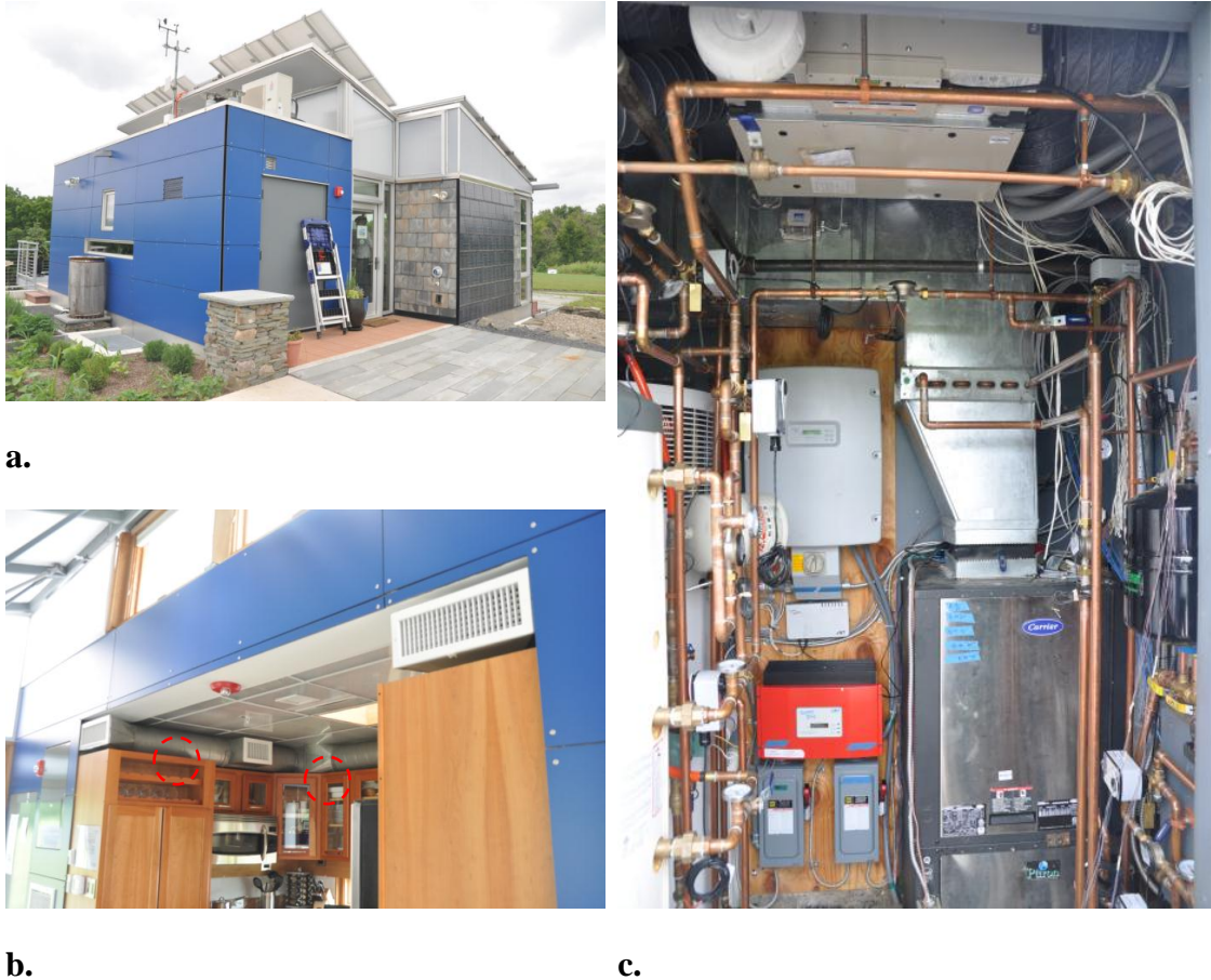
Figure 3. a. MorningStar Solar Home; b. Two of four measurement locations near duct diffusers; c. Packaged unit in mechanical room; red dots are approximate locations for 1/2 in. diameter traverse caps to be installed in the ductwork to enable velocity profiling and to fit particle injection line
