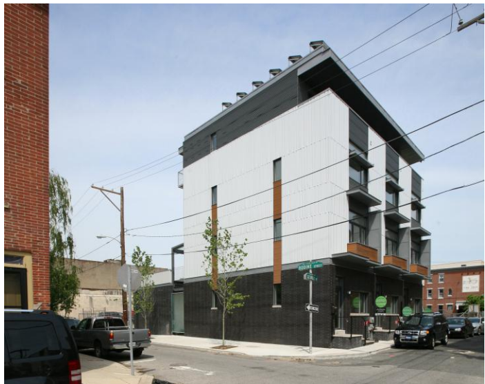
Figure 14: Photo of completed Phase 1 of Stables Townhomes
