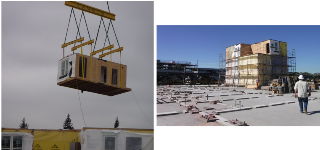
Figure 7. Case Study #1: Lifting and setting units in field
