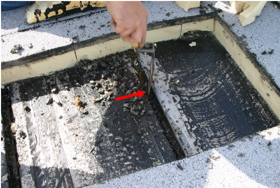
Fig. 13. No grout between joints (arrow) and no topping slab.
