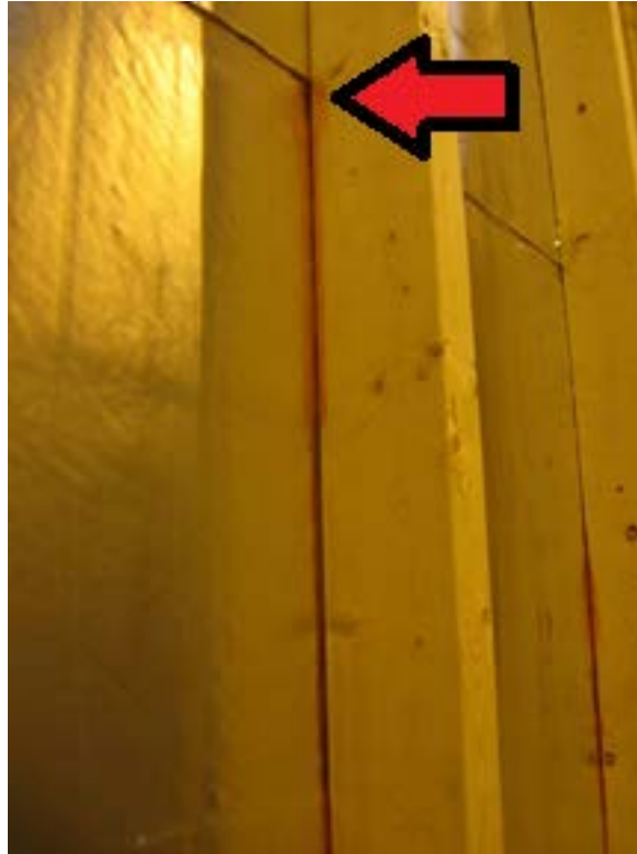
Figure 7. Wall Specimen after Testing with E331 showing water intrusion at foam insulation board taped seams.
