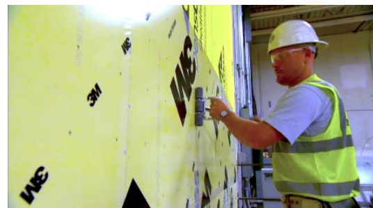
Figure 4 Application of 3M™ barrier (Courtesy of Panthereast)
