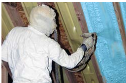
Figure 25 Application of STYROFOAM™ Brand Spray Polyurethane Foam (Courtesy of The Dow Chemical Company |dowbuildingsolutions.com)
