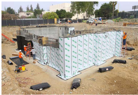
Figure 13 Installations of MEL-ROL Membranes (Courtesy of W. R. Meadows, Inc.)
