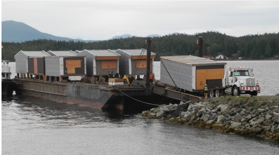
Figure 14. Case Study #2: All six sides of modular units were wrapped with WRB and temporary roofing membranes
