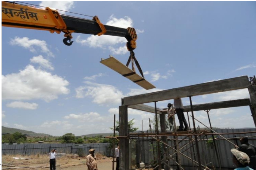
Figure 2. Erection of Ferrocement member
