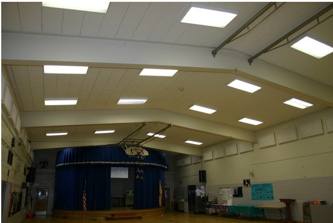
Fig. 7. Roof of school gymnasium constructed using assembly concrete blocks.
