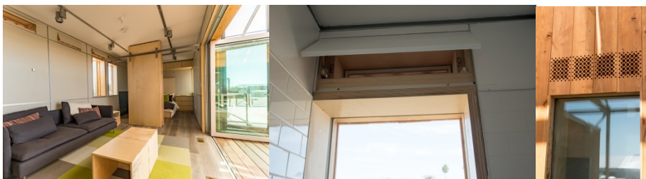
Figures 17-19: Photographs showing the integration of ventilators with interior finishes, a close-up of one ventilator showing interior operable door, a close-up of one ventilator showing exterior perforations.
