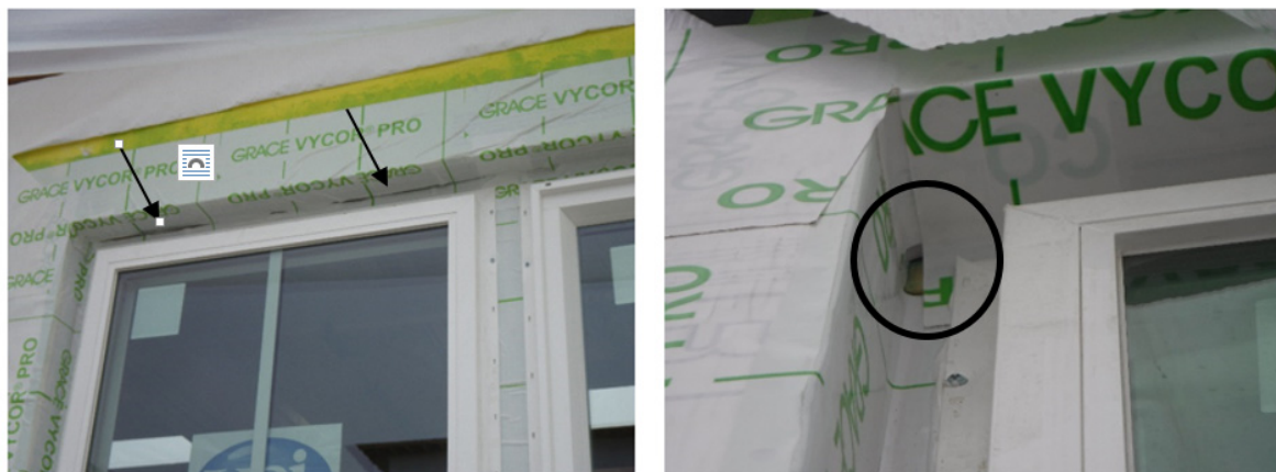
Figure 8. Case Study #1: Defects in the factory installed window flashing included cuts in the membrane, tenting, and gaps that had to be field corrected
