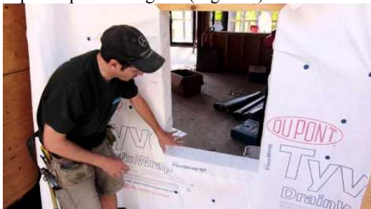
Figure 3 Application of DuPont™ barrier (Courtesy of Professional Remodeler magazine/Photo: Erika Taylor)
