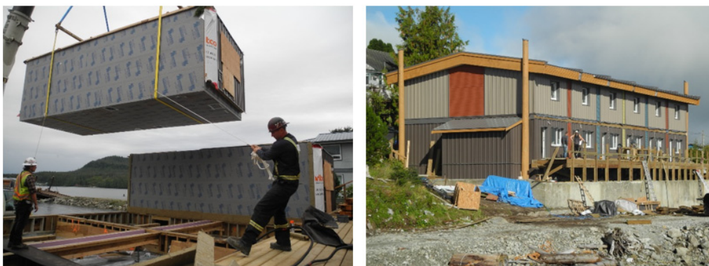
Figure 16. Case Study #2: Placement of modules and photo of near complete project
