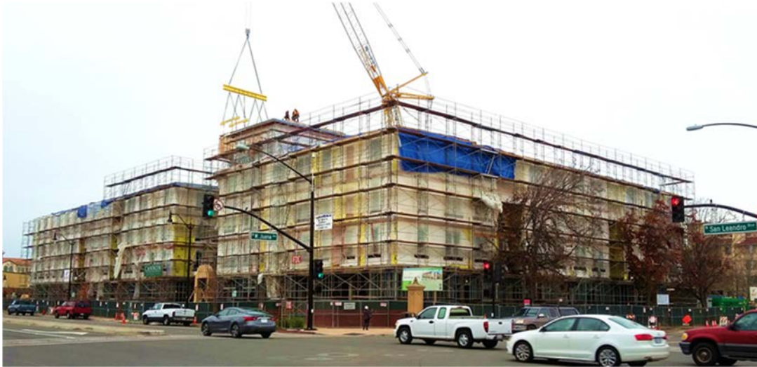
Figure 4. Case Study #1: During construction
