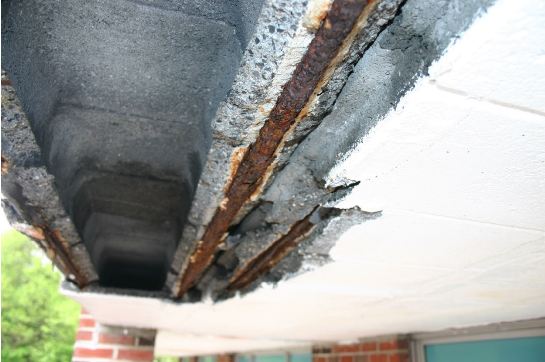
Fig. 10. Spalled concrete cover with exposed reinforcement.
