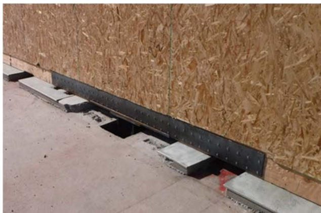
Figure 11. Case Study #1: Misaligned pipe penetrations through slab and curbs Temporary Rain Protection
