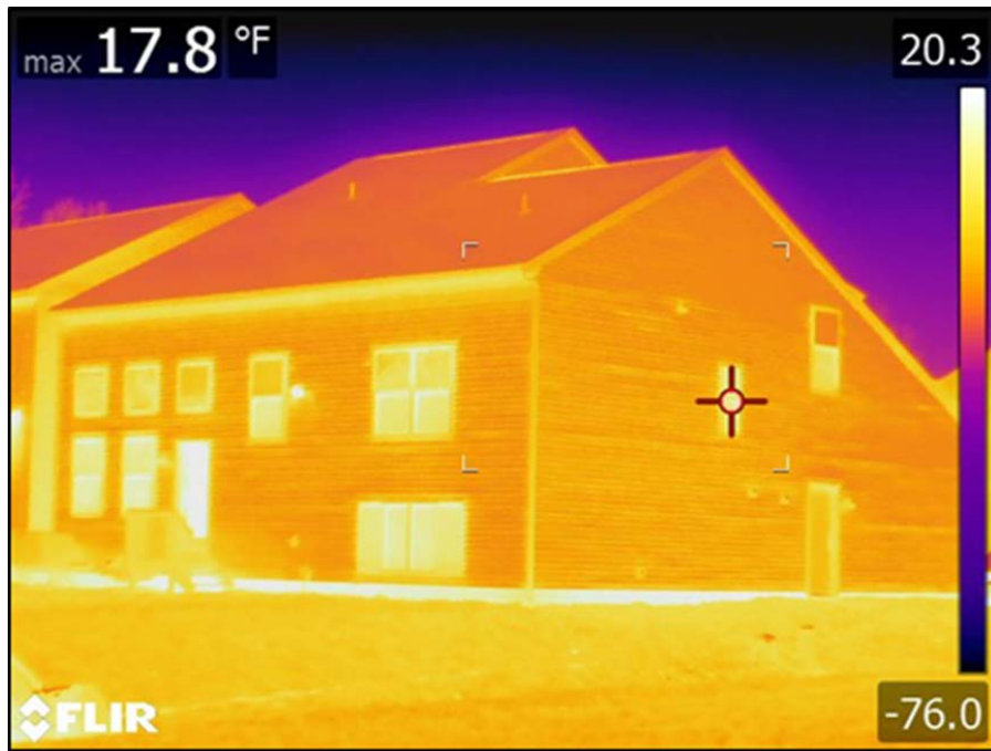
Figure 5. IR Photography of house in Columbus, OH with exterior continuous insulation.
