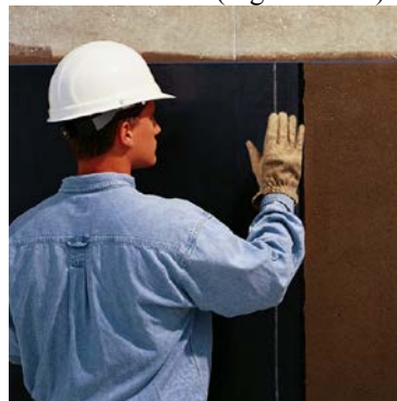
Figure 12 Application of TAMKO®TW-60 Sheet (Courtesy of TAMKO)
