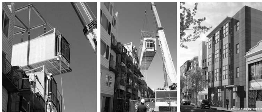
Figure 1. SoMa Studios, a 23-unit apartment building in San Francisco’s trendy South Market district (image by Modular Building Institute (MBI)).
