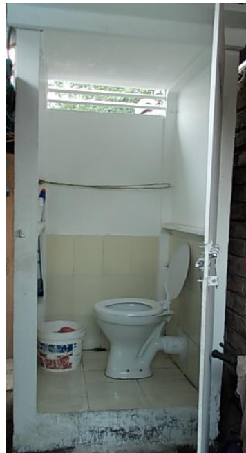
b) Toilet installed in slum
