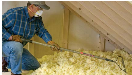
Figure 19 Application of UltraTherm™ Fiber Glass (Courtesy of Cerainteed)
