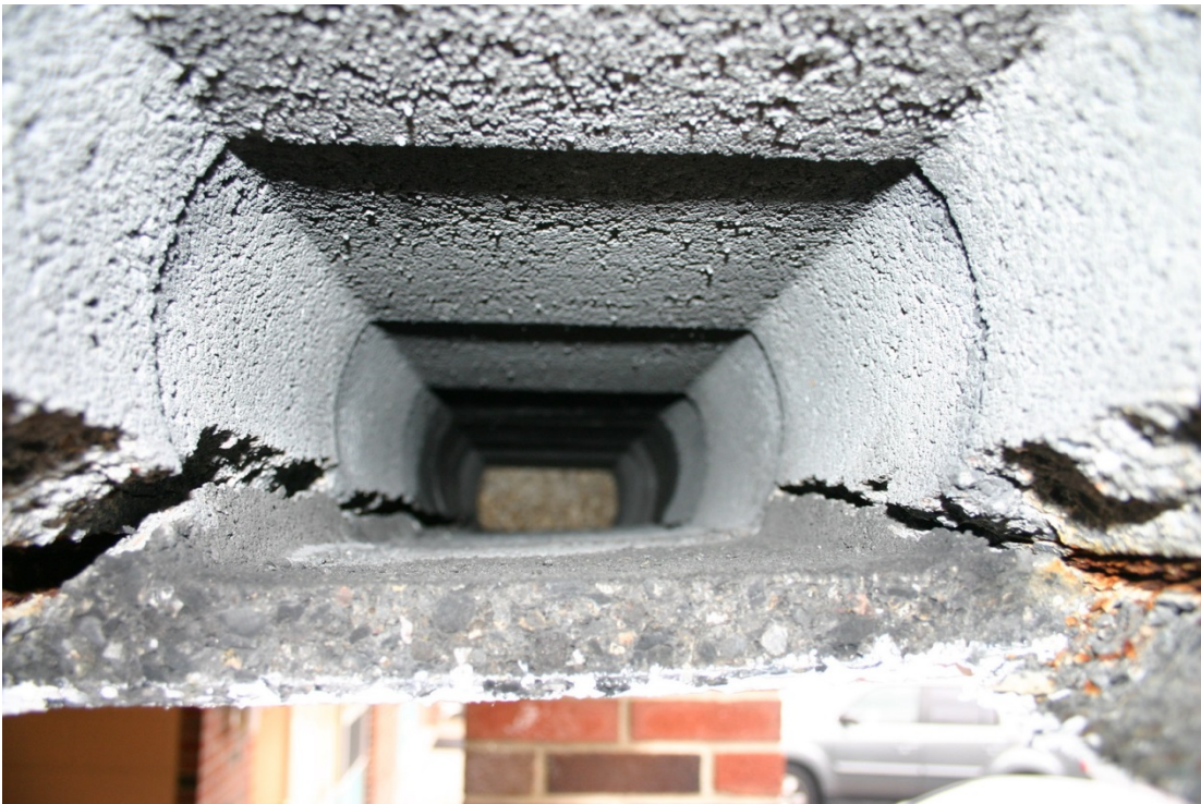
Fig. 9. Cracks viewed from within the hollow core.
