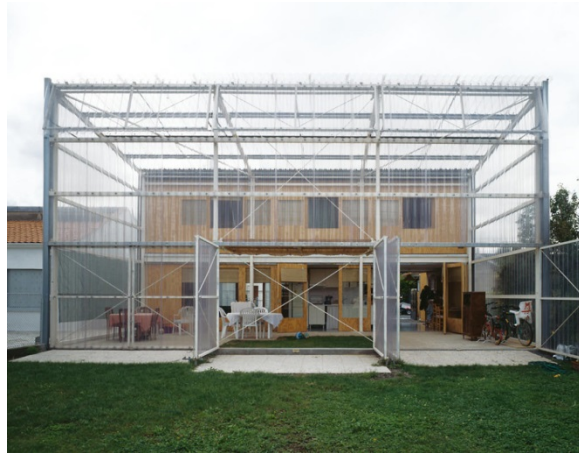
Figure 4: Lacaton & Vassal's Latapie House, which features an elegantly detailed polycarbonate enclosure outside the main conditioned volume.
