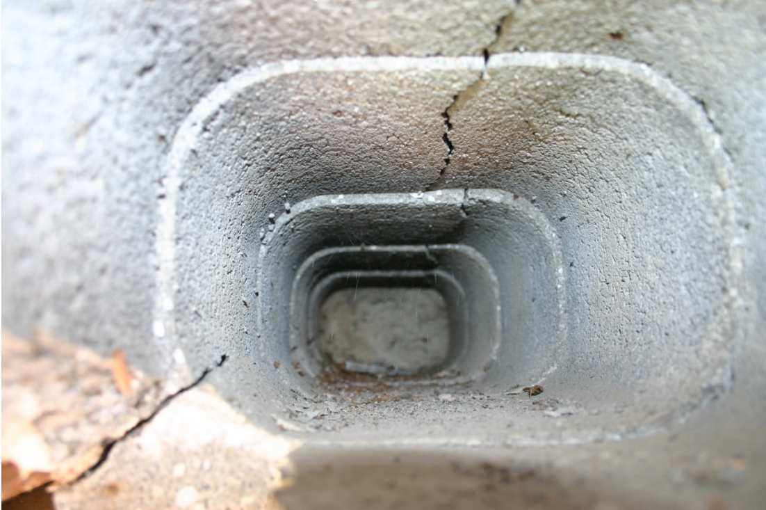
Fig. 8. Cracks viewed from within the hollow core.
