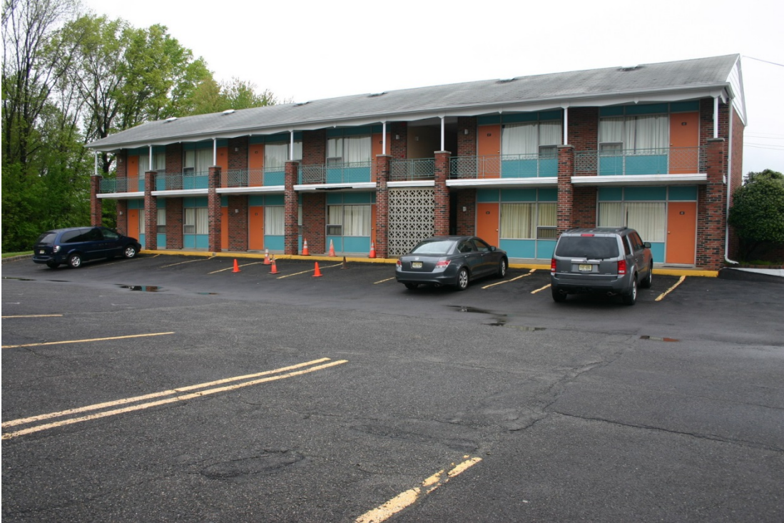
Fig. 4. Floors and balconies constructed using assembled concrete blocks.
