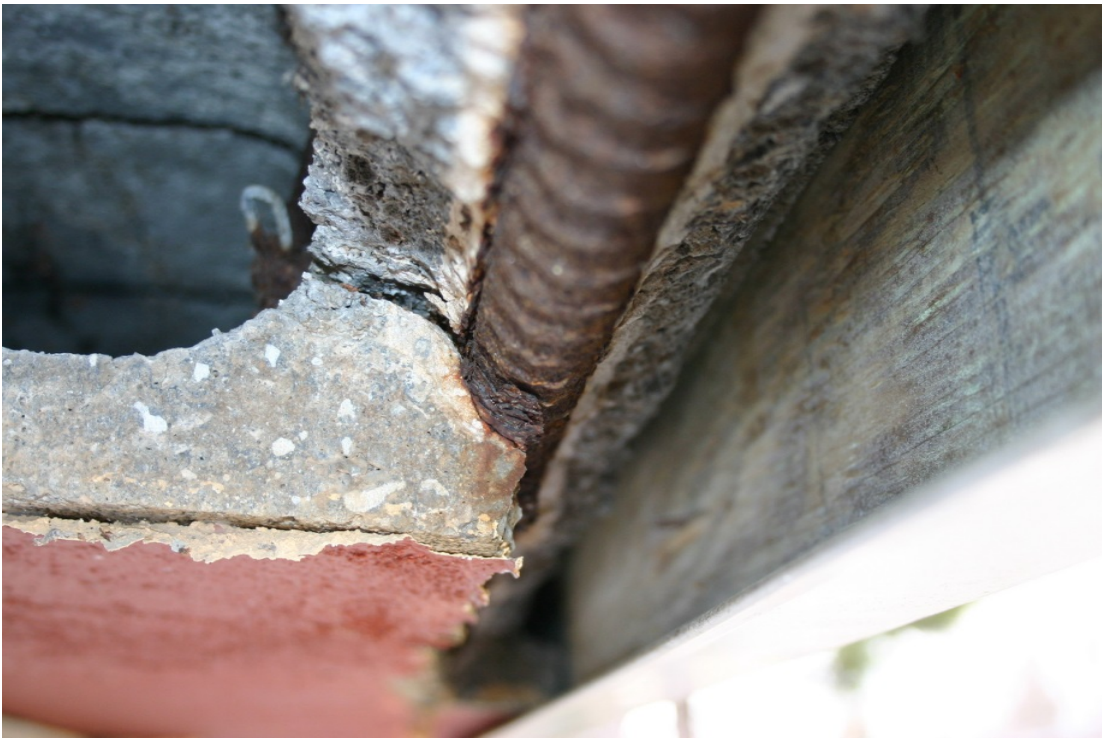
Fig. 11. Close-up of corrosion and section loss on exposed reinforcement.
