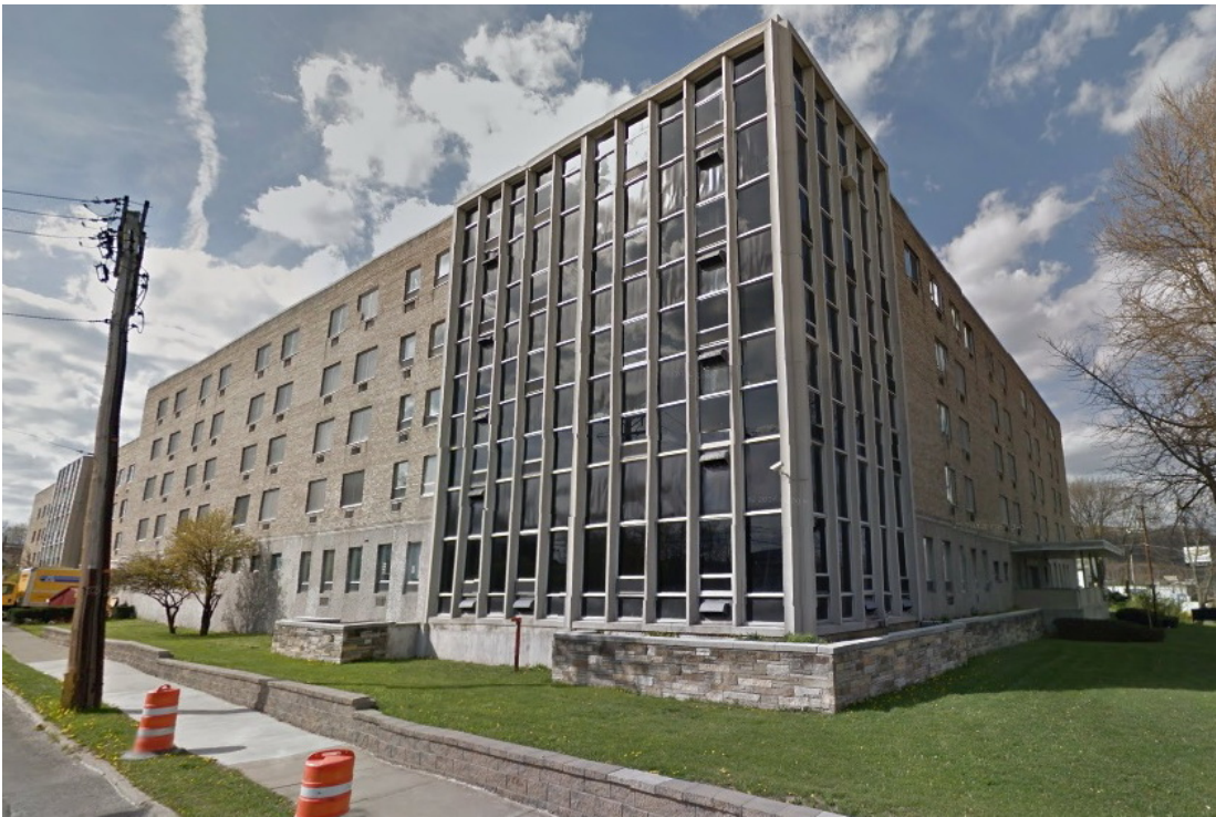
Fig. 5. Floors of nursing home constructed using assembled concrete blocks.
