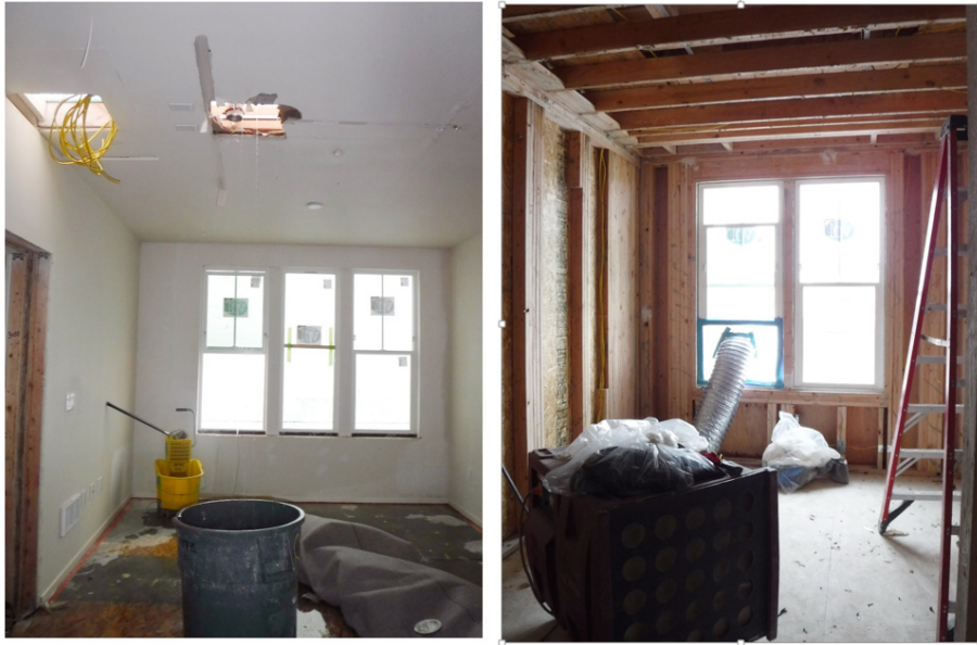
Figure 12. Case Study #1: Water intrusion during construction required extensive removal of interior finishes
