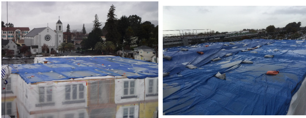
Figure 13. Case Study #1: Improved temporary rain protection during construction
