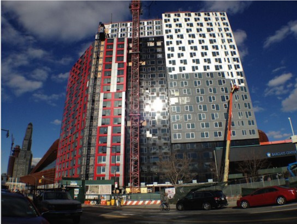
Figure 3. Atlantic Yards Building 2, 33 story modular high rise project in Brooklyn, NY
