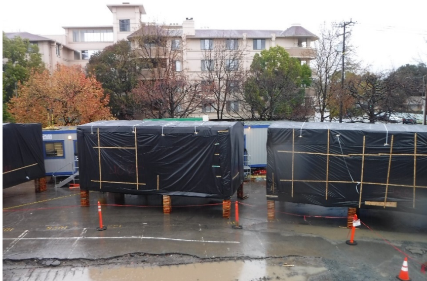
Figure 10. Case Study #1: Despite being wrapped in plastic, heavy rains resulted in water damage to some units during transport
