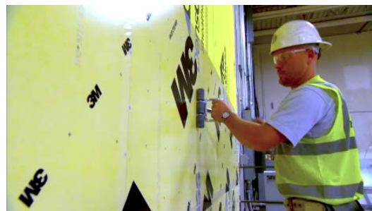
Figure 4 Application of 3M™ barrier (Courtesy of Panthereast)
