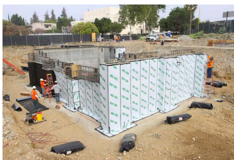
Figure 13 Installations of MEL-ROL Membranes (Courtesy of W. R. Meadows, Inc.)
