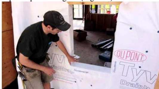
Figure 3 Application of DuPont™ barrier (Courtesy of Professional Remodeler magazine/Photo: Erika Taylor)
