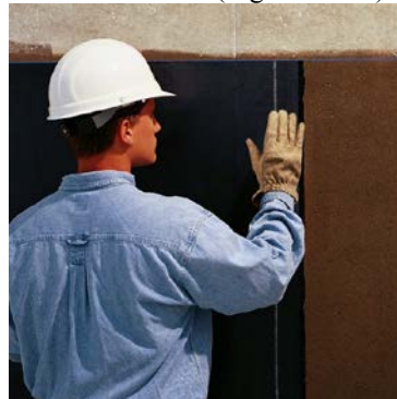
Figure 12 Application of TAMKO®TW-60 Sheet (Courtesy of TAMKO)
