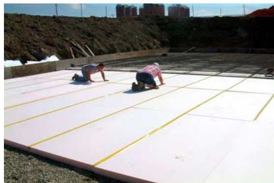
Figure 21 Installation of ThermalStar® X-Grade (Courtesy of Altas EPS)
