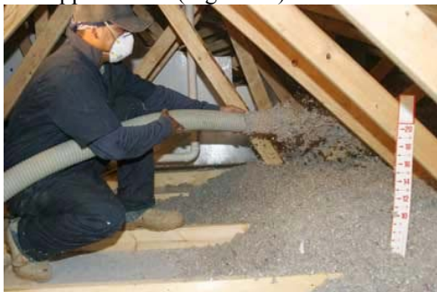
Figure 18 Application of UltraTouch™ Cellulose
