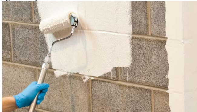
Figure 16 Application of DuPont™ Tyvek® Fluid Applied WB (Courtesy of DuPont)
