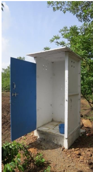
a) Toilet installed in farm
