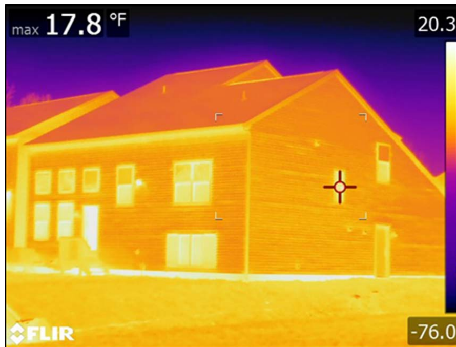
Figure 5. IR Photography of house in Columbus, OH with exterior continuous insulation.
