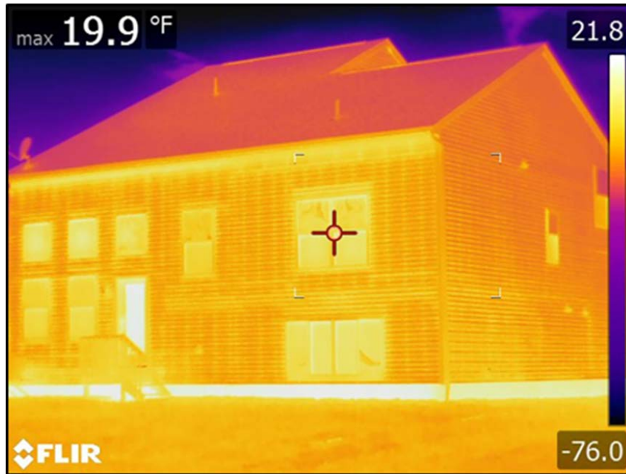
Figure 4. IR Photography of house in Columbus, OH with no exterior insulation.
