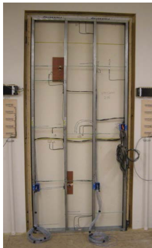
Light Gage Steel Framing
