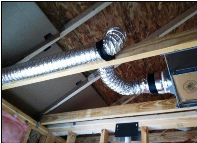
Figure 2: Excessive turns in duct line.
