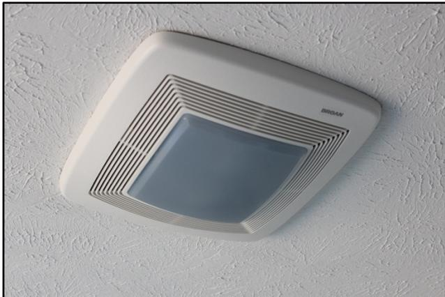
Figure 1: Exhaust only mechanical ventilation.
