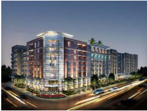
Gables Tanglewood, Houston, Texas. In-progress
