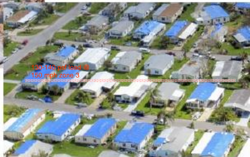
Houses with damaged or missing roof sheathing in Florida
