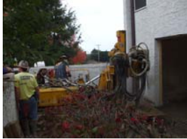
Installing Micropiles
