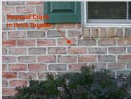
Differential Settlement From Poor Fill Materials
