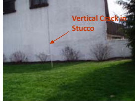
Differential Settlement From Bearing on Fill Materials
