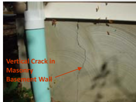
Differential Settlement From Poor Fill Materials
