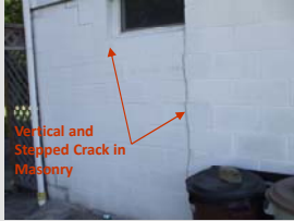
Differential Settlement From Possible Sinkhole Activity
