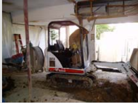
Preparing to Underpin
