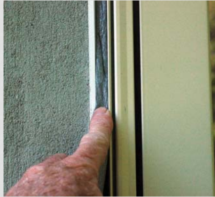
Backer Rod Inserted
