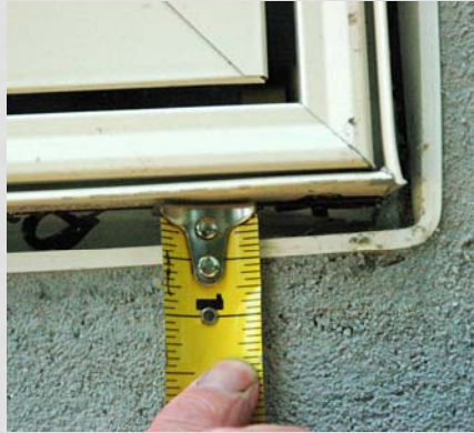
Casing Bead Installed
