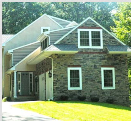
Adhered Masonry Veneer
