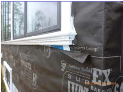
Courtesy of William Dare (Spotlight Home Inspection, LLC)
