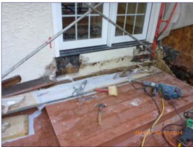
Courtesy of William Dare (Spotlight Home Inspection, LLC)
