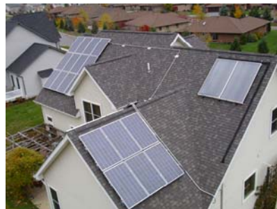
5.5 kw PV system and solar water heater by Envinity in State College
